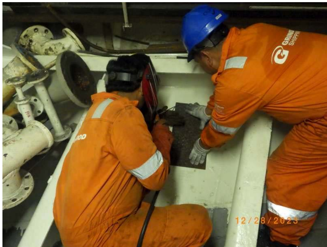
TEMPORARY REPAIR OF THE DAMAGE AREA
