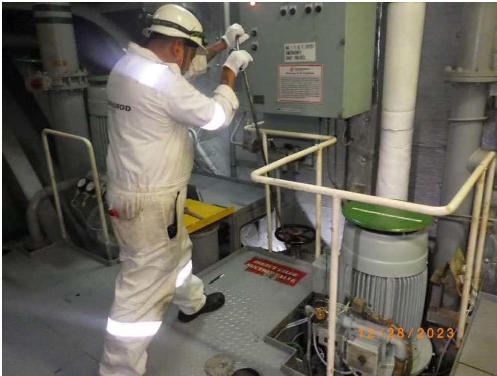
OPENING THE EMERGENCY BILGE SUCTION VALVE
